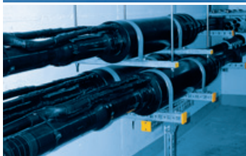
Laying in a tunnel. Joints with Cu-tube and HDPE-coating in a tunnel.
