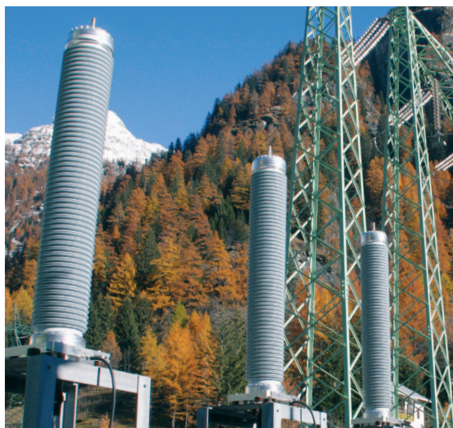
Installed explosion resistant termination at 245 kV level.
